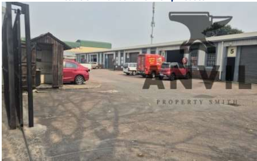
Picture 6: Spring Field Industrial Park
